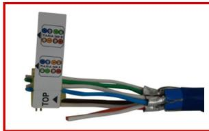
Cut two pairs short by ca. 10 mm. Insert the shortened pairs.
